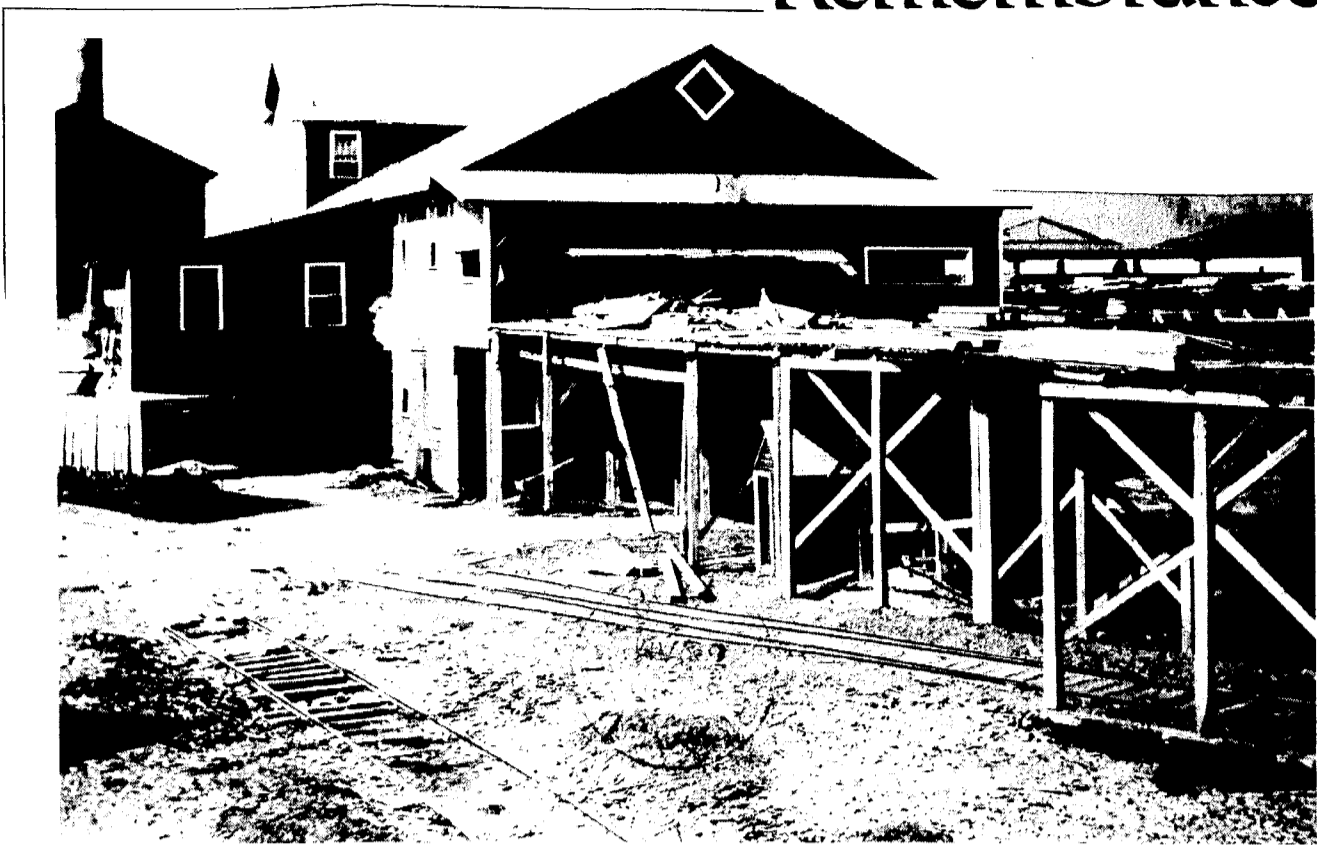
This view of the VanPlaten lumber mill, which was located in the north Boyne area of town, shows how high the scaffolding was that the workers took the lumber off of to stack on the ground for drying. The freshly cut lumber was pushed on small railcars out to the drying areas by the workers. The railroad tracks on the ground were for the incoming lumber that was cut from the hills around the area and brought to the mill for cutting by train. If you have any pictures of the early days that you would like to share with our readers, bring them in and we'll copy them.
