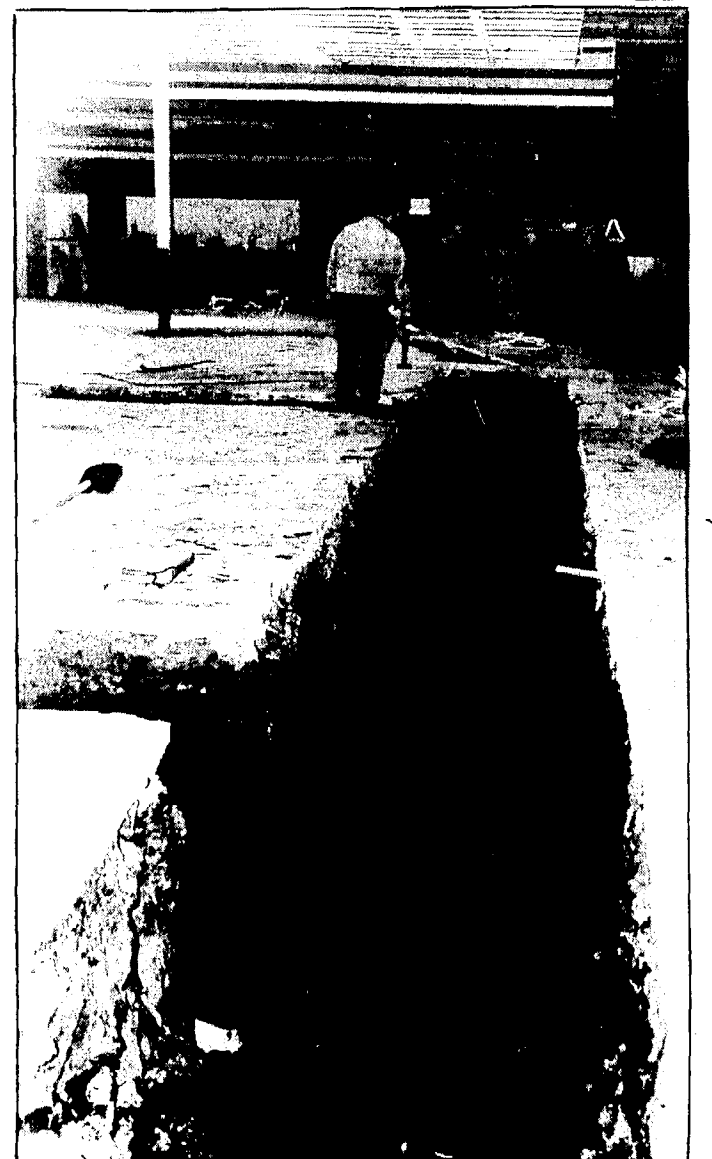
Work on the new Glen's Market that is coming to Boyne City is progressing on schedule, according to the contractors who have started the work on May first. The store is expecting to have all the work completed in time for the Fourth of July celebration. The contractors have had to install trenches in the floor of the old Country Star building to accommodate the new refrigeration piping in the supermarket.
