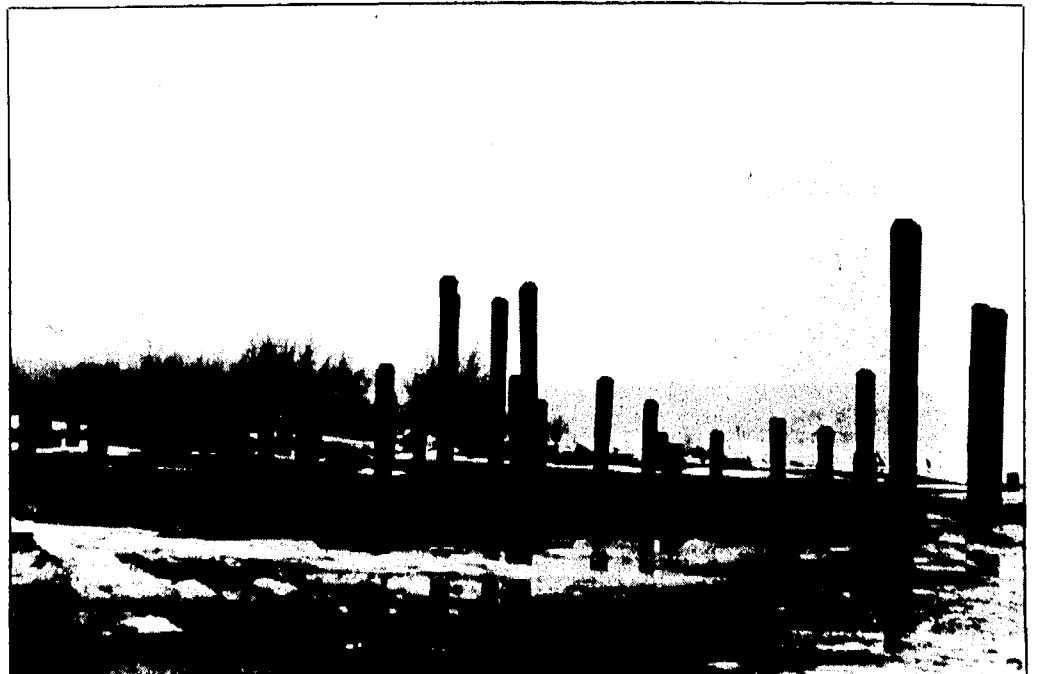
"Just three or four nice warm days," said one of the developers, Rick Smith, "And we'll be able to start building One Water Street." The project, which in the first stage includes a restaurant on the waterfront, will see the pilings get cut flush with the ground perhaps as early as
