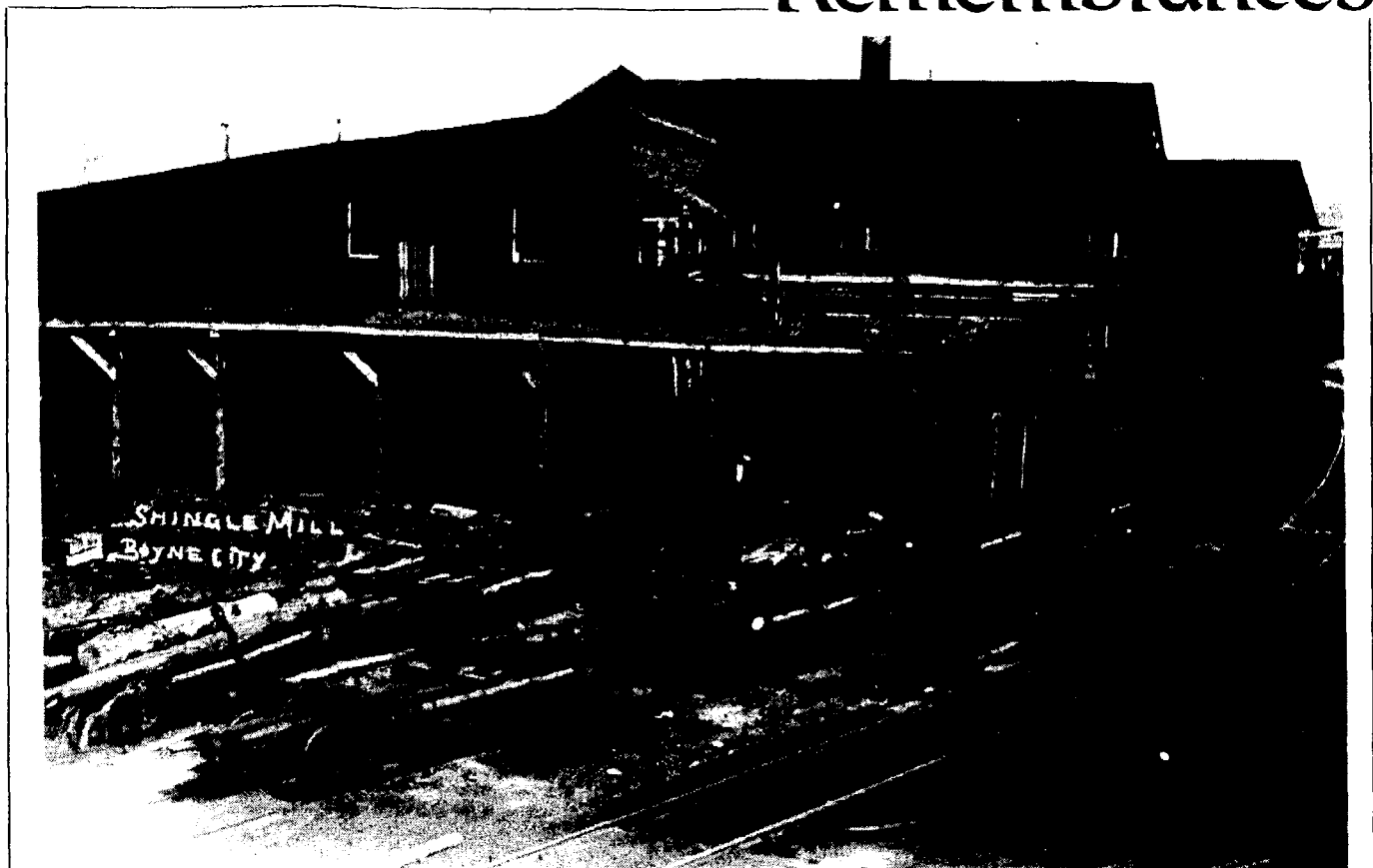
Located on the waterfront behind the stores along S. Lake Street and next to the old railroad roundhouse was the White & Co. Shingle Mill. The mill split cedar into shakes for many houses in Chicago and other parts of the nation that could be reached by water. All the carts with the railroad type wheels were used to take the lumber after it was cut out to the drying racks.
