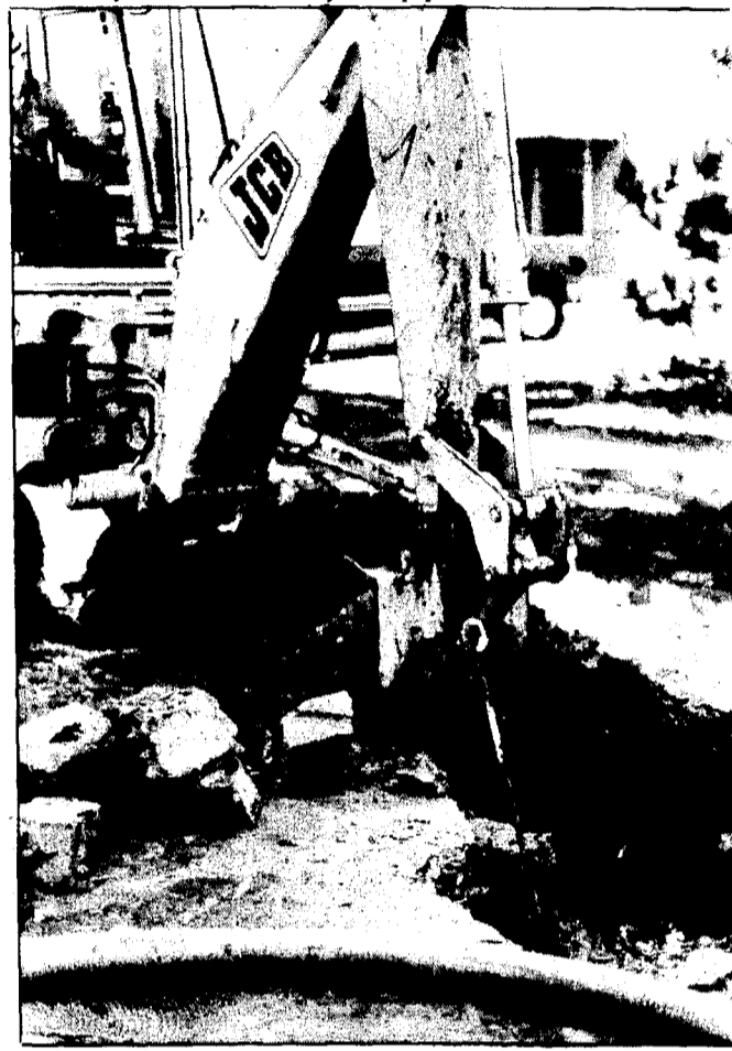
City workmen worked desperately to fix a water main break Tuesday afternoon. The break left much of the north side of town without water after officials had to shut it down to fix the leak. Leaking water from the break shorted out underground electric lines that forced the closing of Bendix/Courter's second and third shifts.
