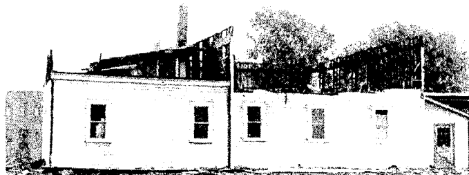
Although construction people are working hard to beat the weather on building, others are in the process of beating the weather in tearing down, as this crew is working on the old Eagles Hall here in Boyne City. The tearing down of a building is probably harder than the construction of it when it was new.
