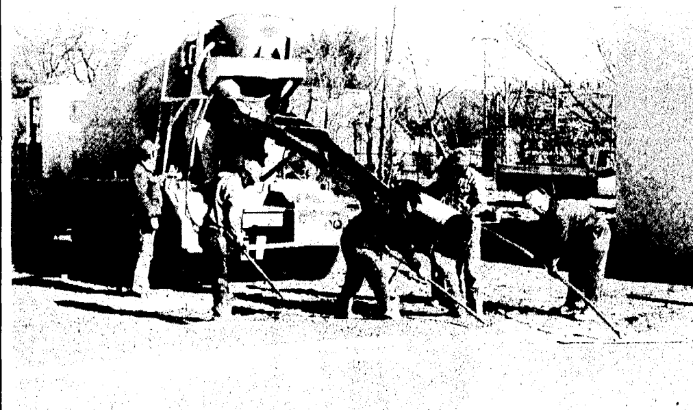
Working to beat the annual freeze up, these cement finishers are laying the floor to the new Boyne Auto Store which will be located behind the post office on East Street. The construction is hoped to be completed by Christmas according to a store official.
