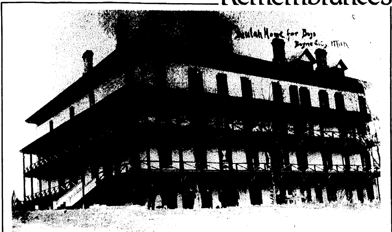
While it ended up as the Beulah Home for Boys, this structure which was built back in the early 1800s, started off as H.B. Chapman's Hotel. It was located in the then thriving Bay Springs area which evolved into being called North Boyne. It is now part of the city and the hotel/home was located at the corner of Silver and John Streets. The hotel was built in the hopes that it would attract tourists, then veterans of the Civil War, before being sold in 1904 to become the home for boys. It was run by Herman
