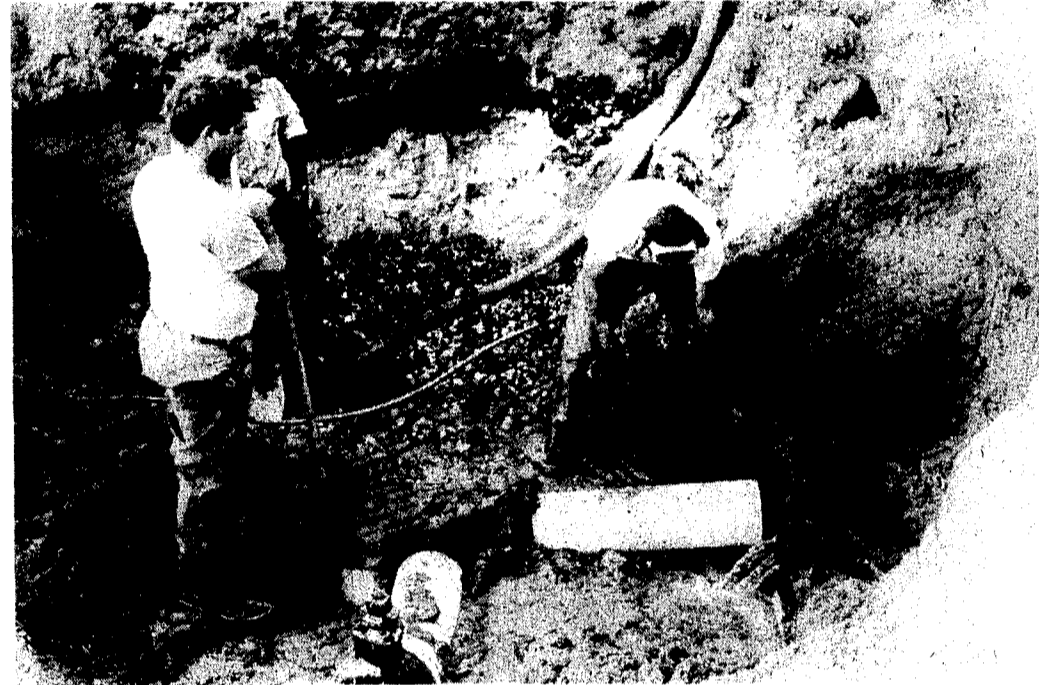
C.H. Smith workers struggle to complete the cutting of the eight inch water main that runs down Lake Street during the changeover to the newly installed water lines that are part of the rebuilding of the street. The underground work for the first block is expected to be completed by this weekend so that the sidewalks and curbing can be poured while the weather is still good. Expected completion for the project is still set for November, although the rains of the last week have delayed the workers a little.
