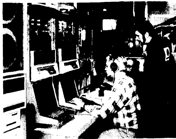
Technicians from a division of Rockwell International operate a computer console that controls an ultrasonic inspection device inside the Big Rock Point plant's nuclear reactor. Results of an inspection at the plant show that primary piping and the reactor vessel are in excellent condition after 20 years of operation.
