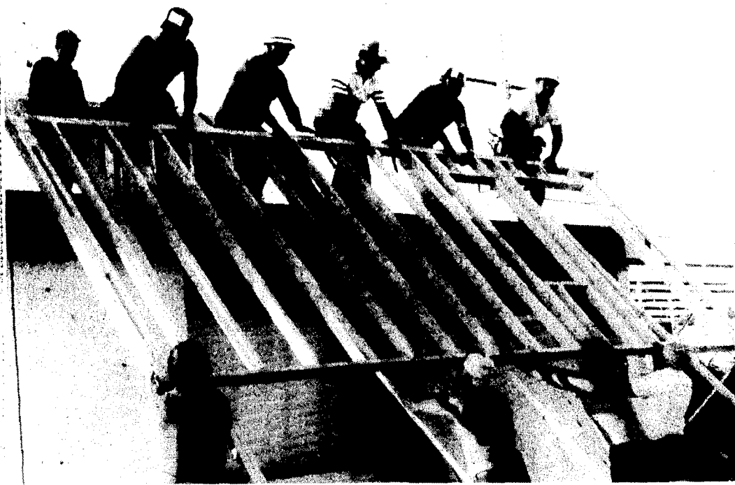
Members of the Boyne City Rotary Club alide one of the walls of the football field press box up and into position last Wednesday. The project was undertaken by the members of the club after it was discovered that the roof was leaking and the floors were getting rotten. One member of the Rotary Club said that Boyne City's new facility will be the best in the north.
