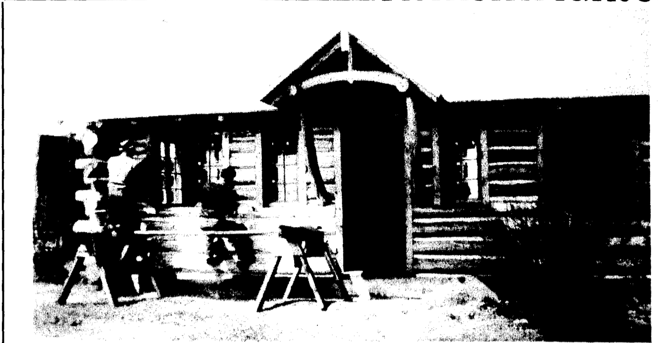
With today's Youth Job Corp bringing back memories to some of the men who helped build this log cabin back in the depression. This picture, courtesy of Art Dobbs, shows the workers of the youth job corp of that era finishing up the work on what is today the office for the Boyne City Chamber of Commerce. Each log had to be caulked and then painted by the members of the corp about
