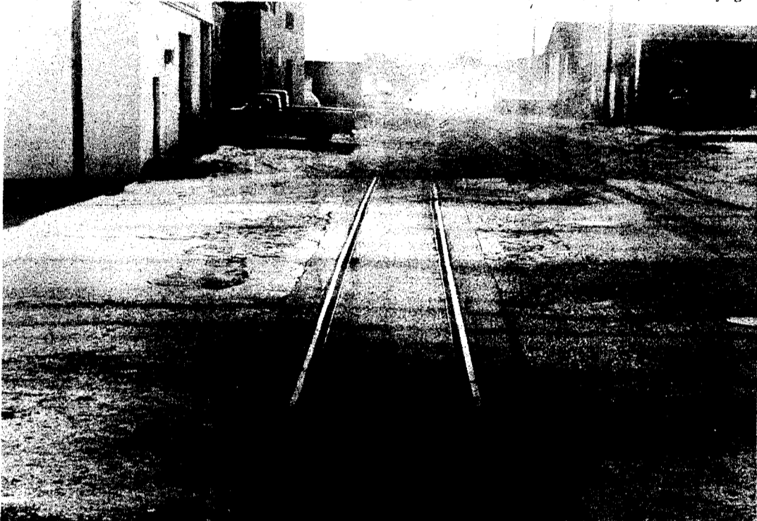
The tracks that cross both Park Street and East Street will be taken up by July 15, according to the recently settled suit that was filed by the city against the Boyne Valley Railroad. In the settlement, the monies will go for the replacing of the
