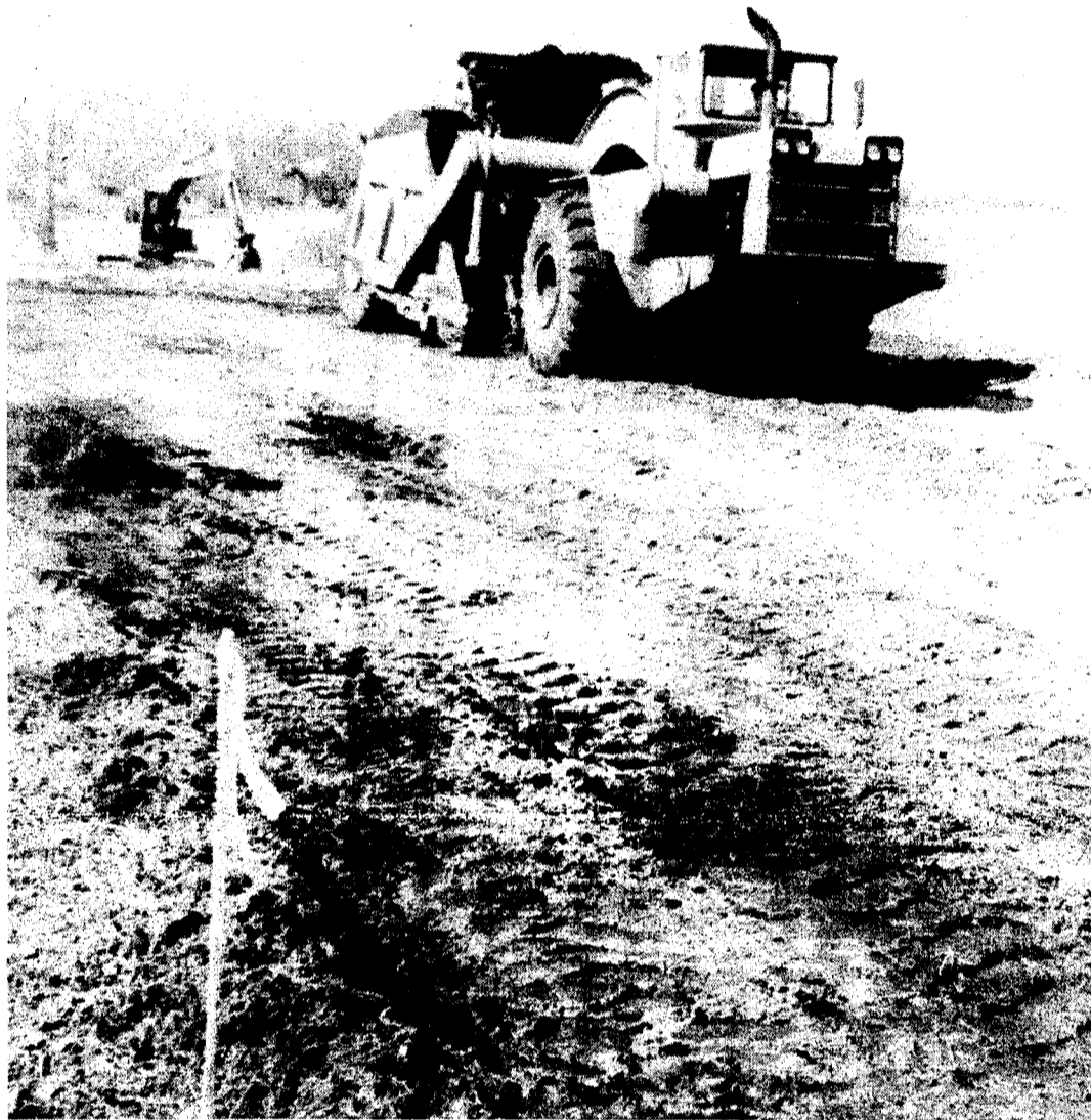
Work was started last week on the new Front Street that was moved along the waterfront on the south side of town. The cost for the new road will be paid by The Harborage, the developer of condominiums between the road and the waterfront. The road will be two lane and will be on higher ground than the present road.
