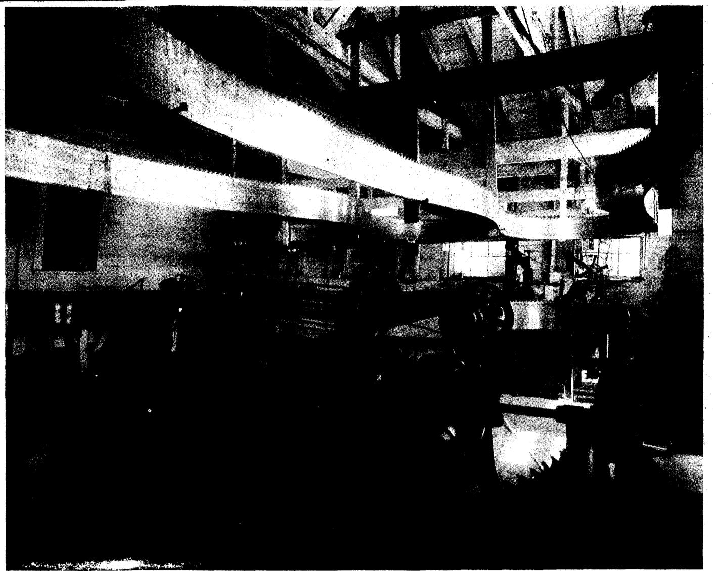
Back in the days of the lumber business in Boyne City, the mills were running ragged trying to cut up all the logs for the many businesses that wanted the virgin White Pine. This picture shows the saw sharpening room at the White Mill No. 3 which was located on the east side of town. The saw blades would be worked for so many hours and then were hand carried by a couple of men down to this room so they could be resharpened. Each blade looks like it was about 40 feet long and ran like a bandsaw. From the picture, it looks like the mill had plenty of blades in case one of them broke or needed replacement. The teeth look like each one was about two inches deep on a new blade, and with each sharpening, got a little smaller in cut. The machinery that sharpened the blades is in the middle of the picture. This was taken in 1918 when the mills were still in operation. The picture was given to us to copy by Ed Hartnell from his collection. He has lived in the area since 1913 and can remember the mills from his childhood.
