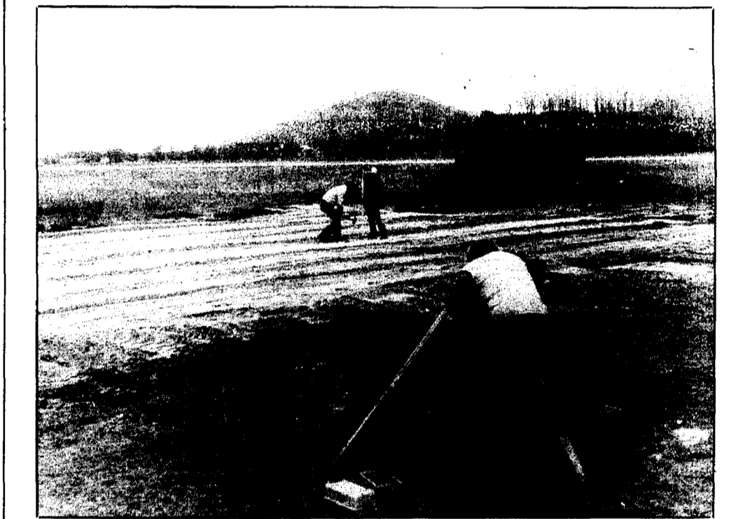
A combination of city workmen and workers from Trumco, the general contractor for the project, have started spotting the footings for the new airplane hangars that will be constructed at the Boyne City Airport. The hangars, being built without city funds by pilots who want to house their
