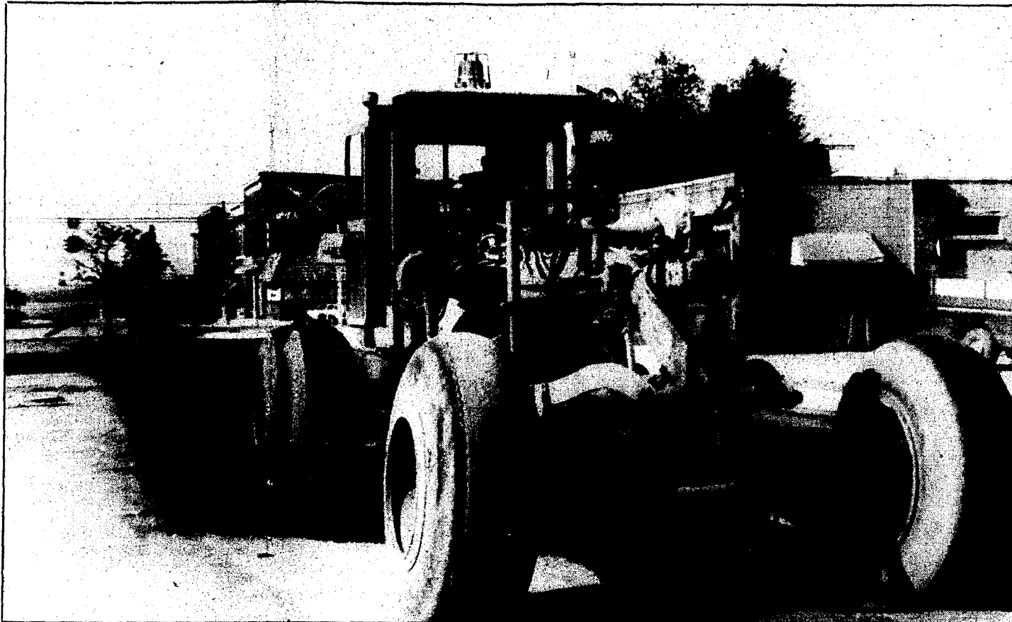
The final grading took place Monday on the Water Street block under construction in preparation for paving on Wednesday. The project is expected to be completed
