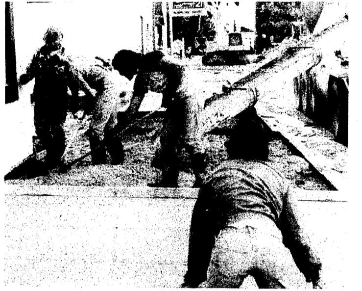
Water Street renovation in Boyne City should be finished by October 23, according to city manager Tim Clifton. Finished, except for the brick paving, he added. Over the last weekend, workers started laying the cement for the sidewalks. The final grading of the street should be done on next Monday or Tuesday and the street will be paved. Clifton added that the work is still ahead of schedule.
