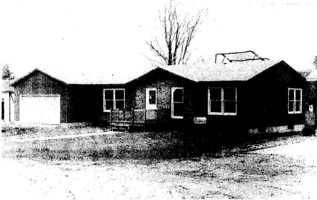
This Spanish design three bedroom home will be open for viewers Oct. 17 and Oct. 18. The house, built by the Boyne City high school's building trades class features a solar hot water system, and has a lot of exceptional construction work done by the students. Instructor Harold Hamlin said
