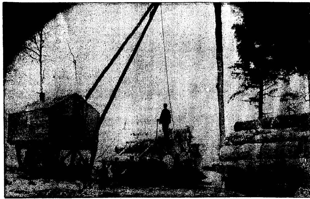
When Boyne City was one of the logging centers of Michigan, the trees were cut farther and farther from town. This meant that the logs would have to be transported by rail to the mill. In this picture, taken during a winter-time about 1910, shows how the logs were piled on the railroad cars. A permanent A frame was set up, and the logs winched up and on to the pile ready to go to the mills. If you have any old pictures of Boyne City and the area around here, and want to share them with our readers, just bring them in and we will see that everyone gets a chance to see Boyne a long time ago.
