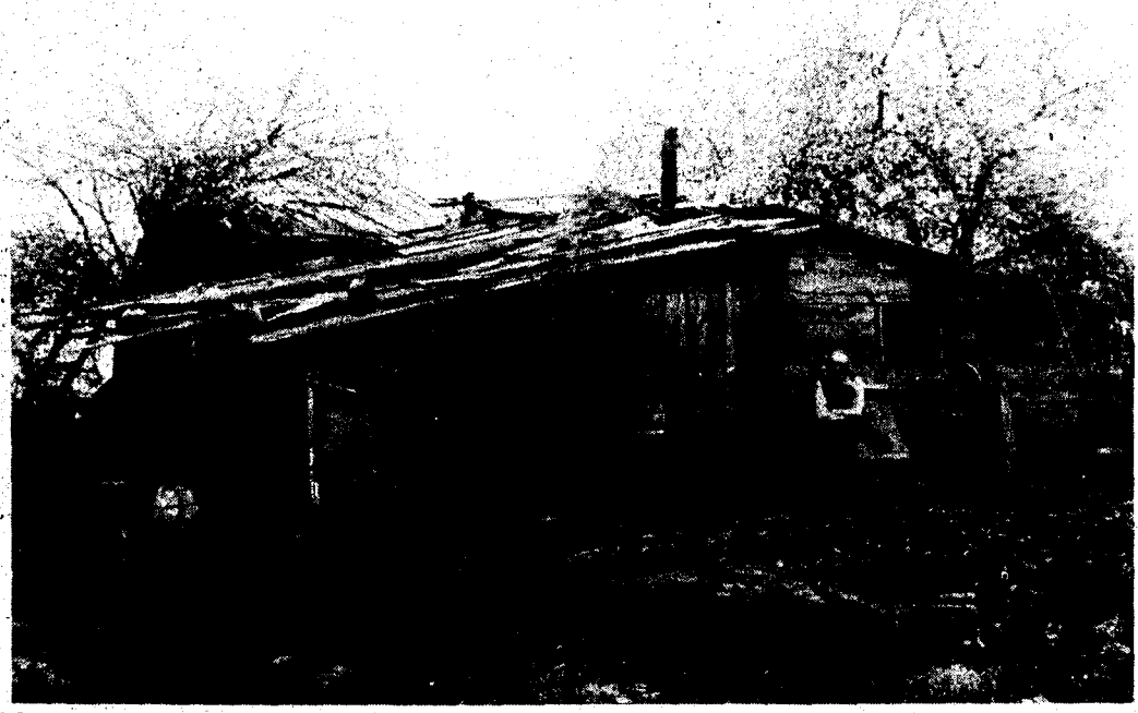
John and Harriet Miller were the first settlers in the Boyne area. They came here on Nov. 14, 1856. This photo shows John Miller sitting in front of their "dream cabin." The photo is from the collection of Bob Morgridge. If you have an old photo from the area you'd like included in Remembrances, drop it off at the Press office, 108 Groveland, Boyne City.
