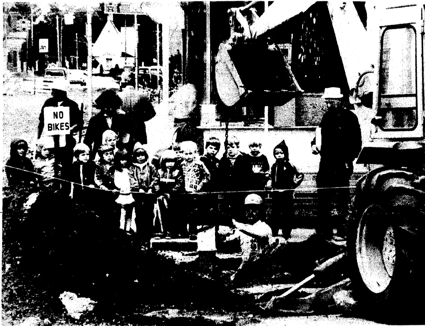
Street construction in downtown Boyne City continues to be a daily "spectator sport" for people of all ages. Youngsters from the Boyne City Nursery Center walked downtown last Wednesday afternoon. They were fascinated with the digging and pipe cutting involved in removing an old fire hydrant from the corner of
