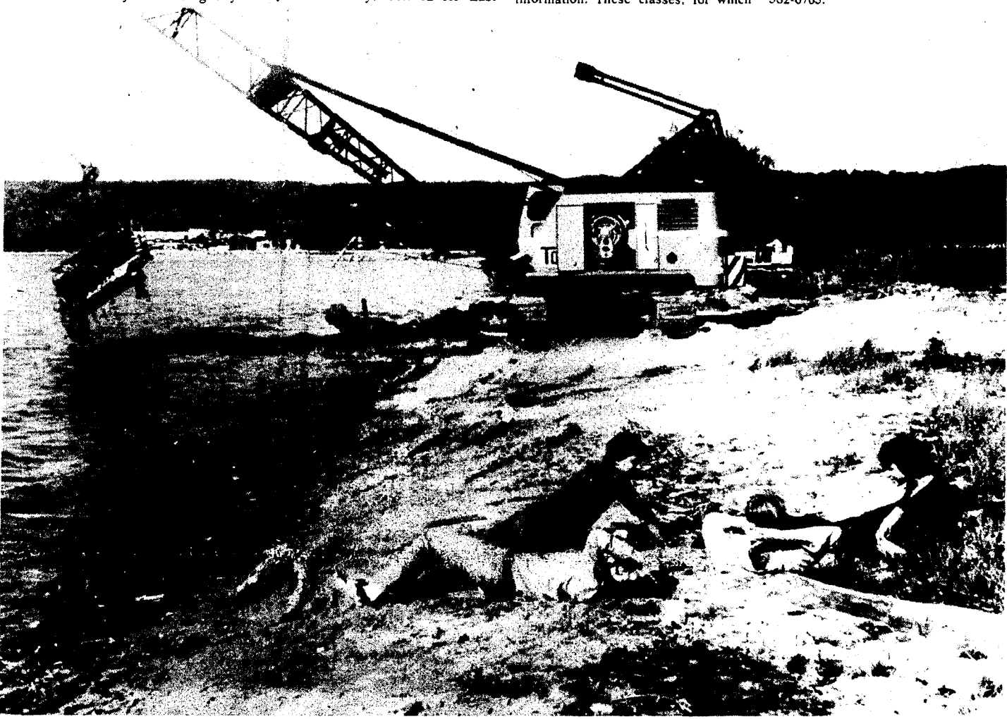
Boyne City's new municipal beach will soon be ready, and these young people can hardly wait. They were watching a crane and bulldozer donated by the Harborage Condominium developers, which were working on the beach last Friday. The crane was dredging debris, left from an old lumber mill, from Lake Charlevoix to make the area near the city sewage treatment plant safe for swimming. About 2,000 cubic yards of sand dredged from the nearby Harborage Marina will be used to fill in the
