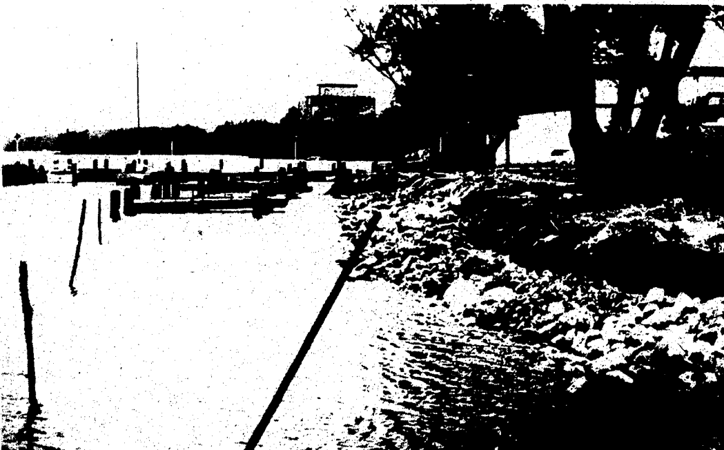
Work is now underway on the shoreline stabilization project at Memorial Park in East Jordan.
