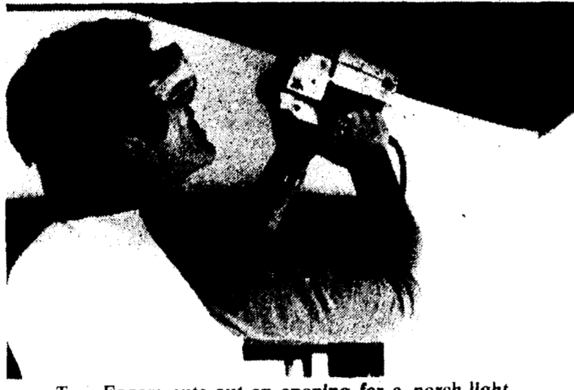
Tom Eggers cuts out an opening for a porch light.
