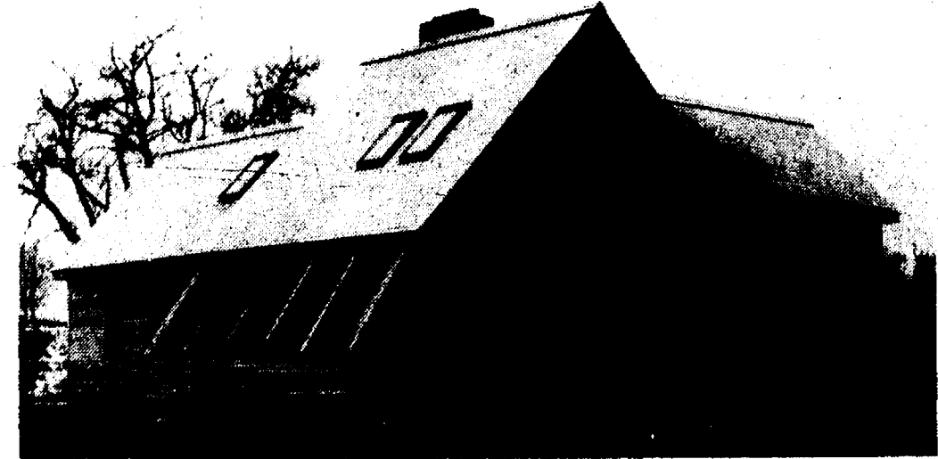
The steep roof line of an old farm house is about all that remains recognizable now that exterior remodeling is nearly complete on Bruce Janssen's home.
