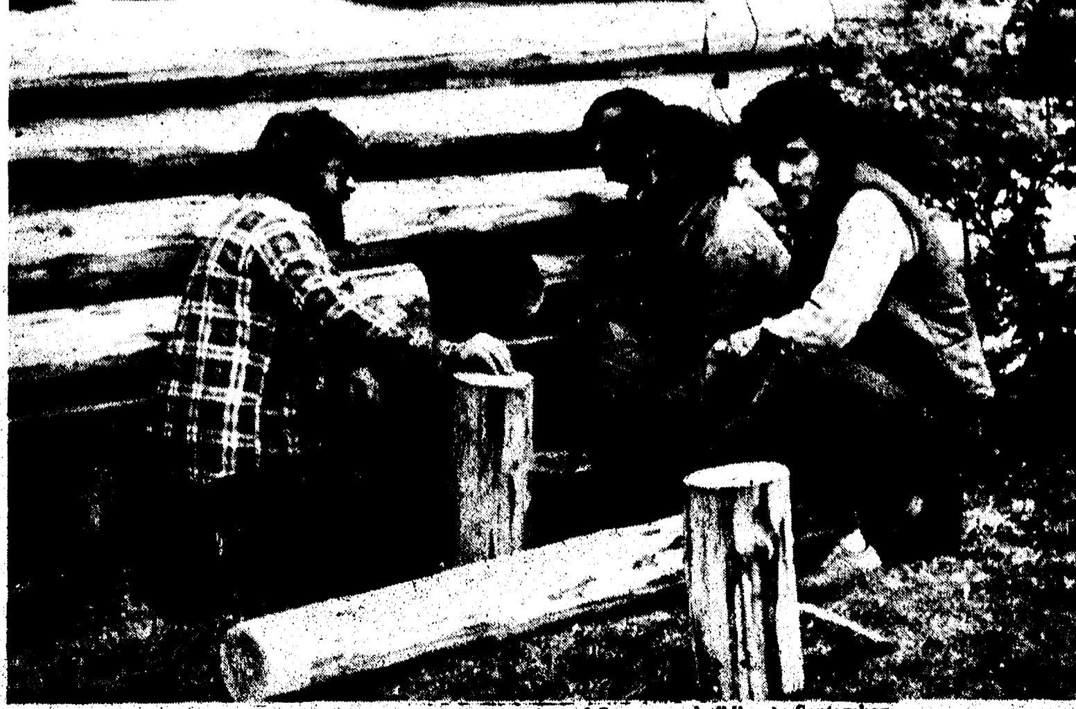
CETA workers renovated the Chamber of Commerce building in September.
