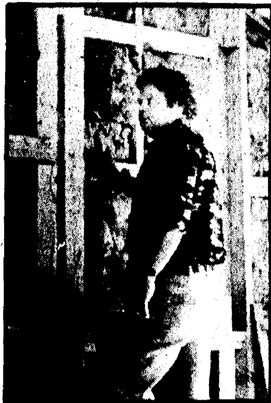
Proper insulation helps cut heat waste and provides more comfortable living conditions. Jack Bohne installing insulation at Wildwood on Walloon.
