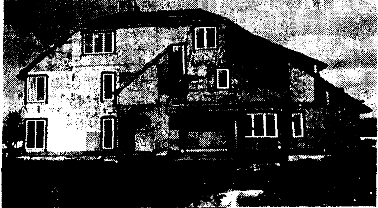
The Harborage—108 units under construction.
