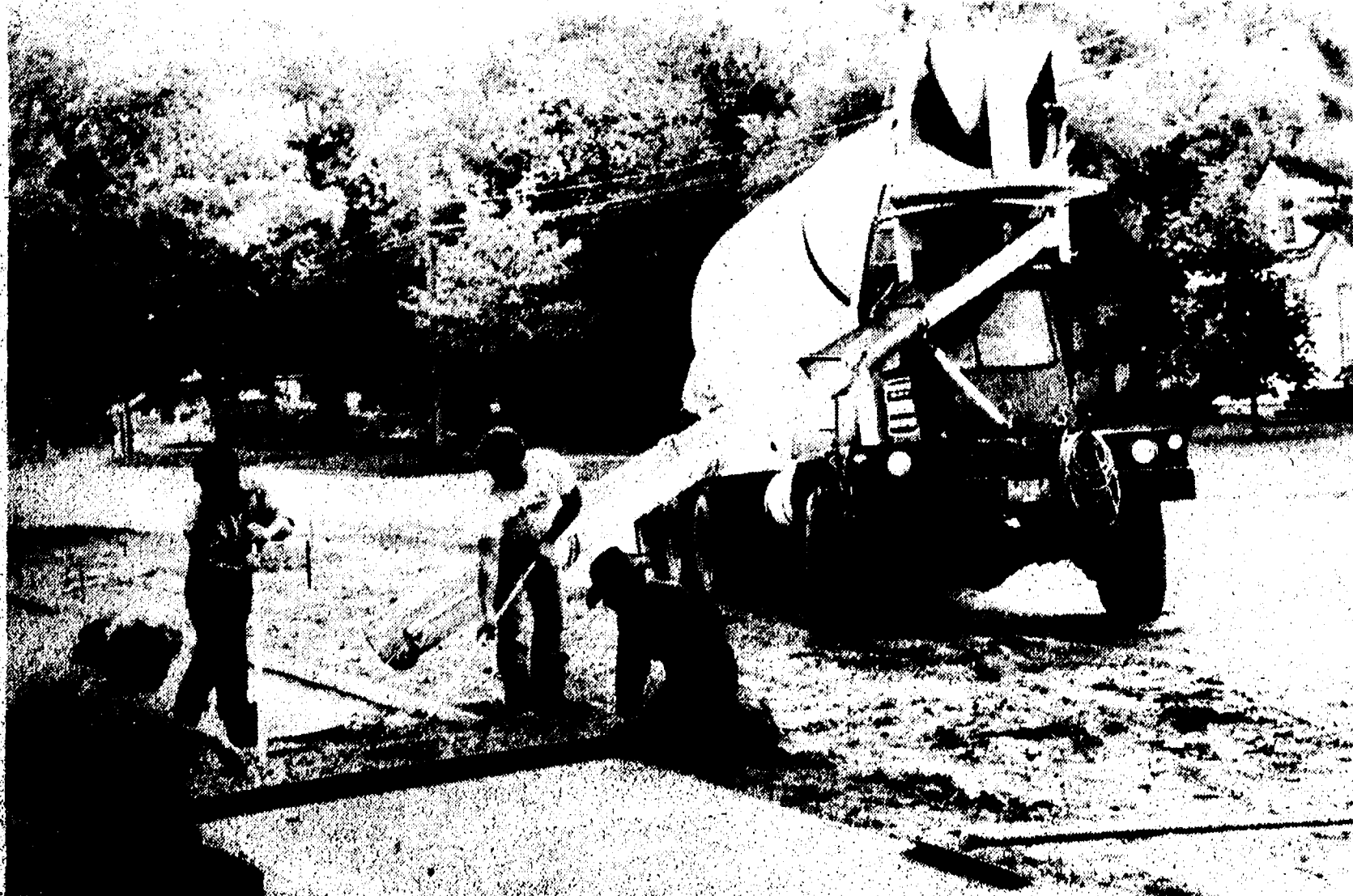
Capital improvements on streets, sewers and sidewalks was a big priority the past year for Boyne City's administration. These construction workers paved 3,000 feet of concrete for sidewalks on the north side of State Street from East to Hannah Street in August.
