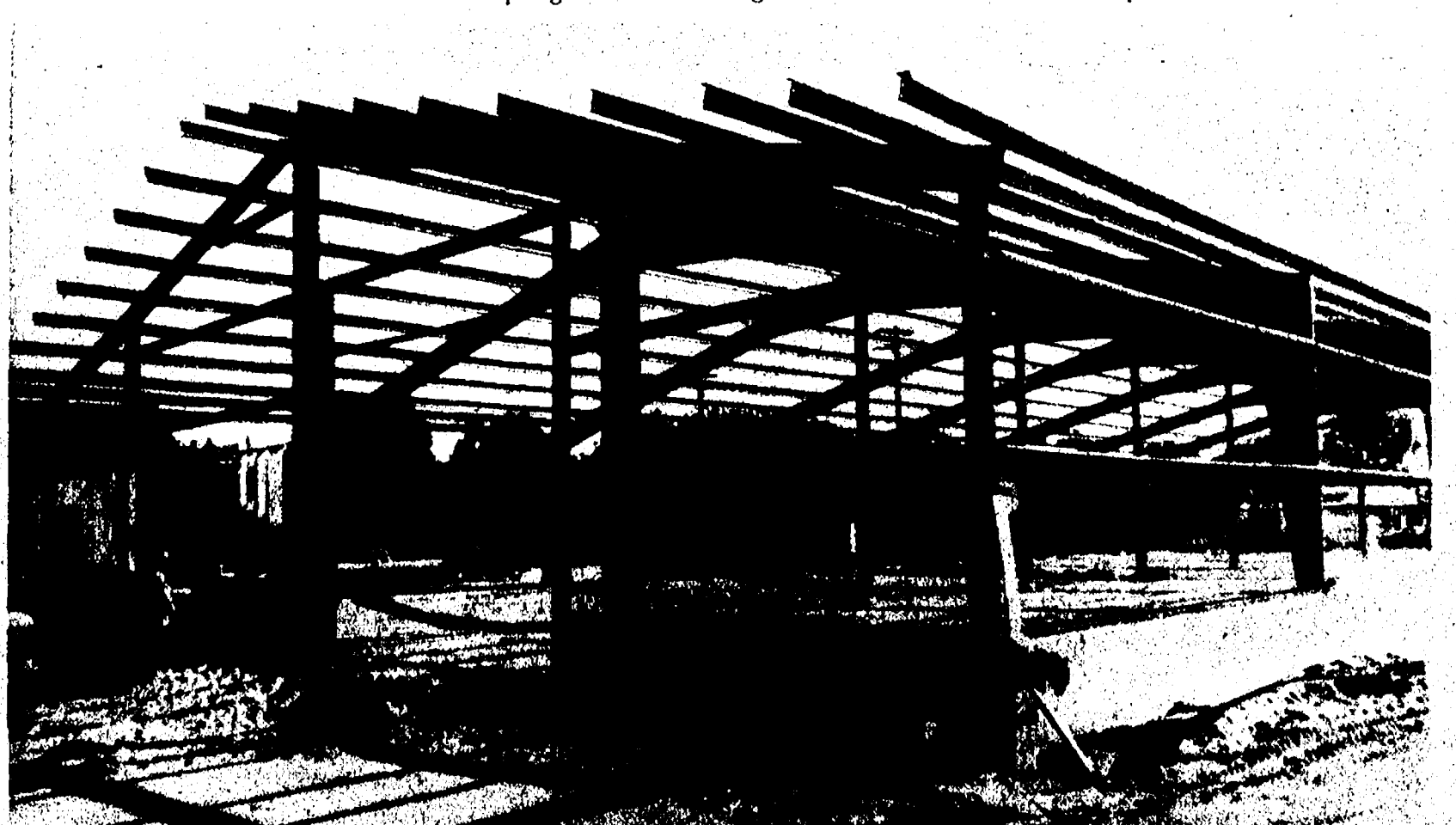
Boyer City's largest construction project in 1979 was restoration of the F.O. Barden & Sons Lumber Co. which was destroyed by fire in May. Construction costs totaled $110,000 for rebuilding the main warehouse.
