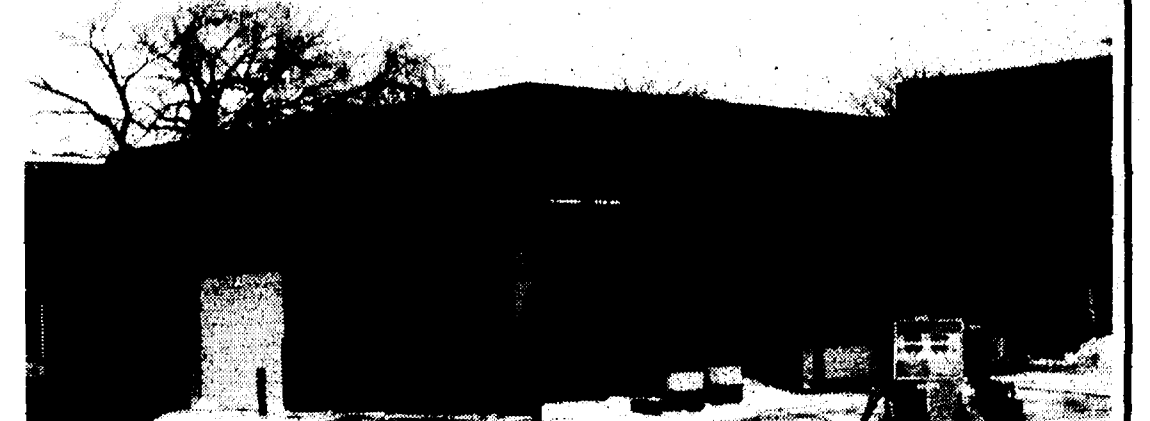
E&M Standard of Boyne City has just completed this service station building after tearing down its old facility. Application has been made for a tax break.
