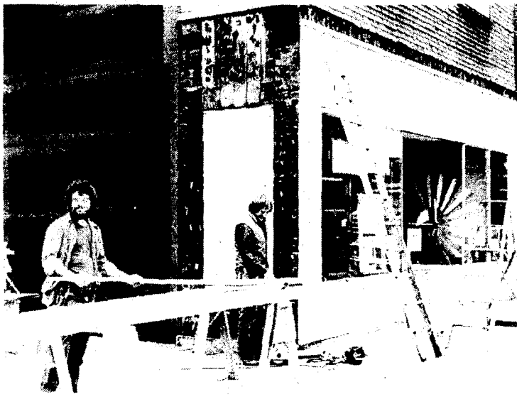
Great Lakes Energy Systems is the first store to start storefront renovations in the city redevelopment plan. Contractor Lee Ekstrom is doing the work.
