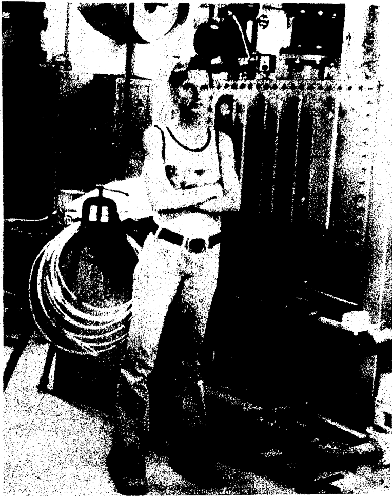
The background may look complicated and it is. It's part of the new heating system for the new East Jordan High School. Diane Haggard, standing in front of this creation, is the lone female to help work with the plumbing systems for the new school.
