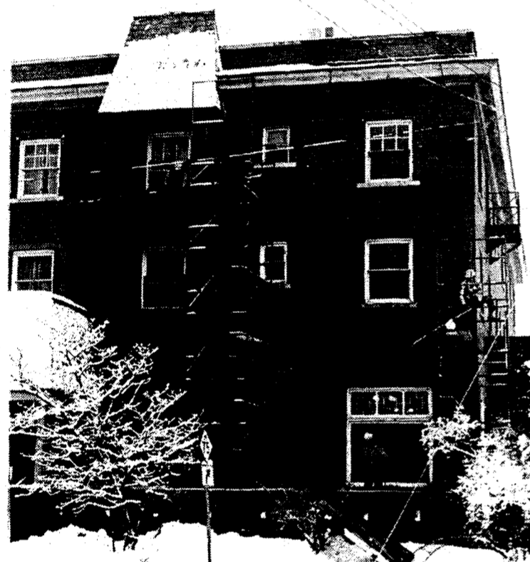
Workers strip off some of the ornamentation from the Dilworth. The new owners want to restore the old hotel to the atmosphere it featured years ago. (Press photo by Neal Colburn).
