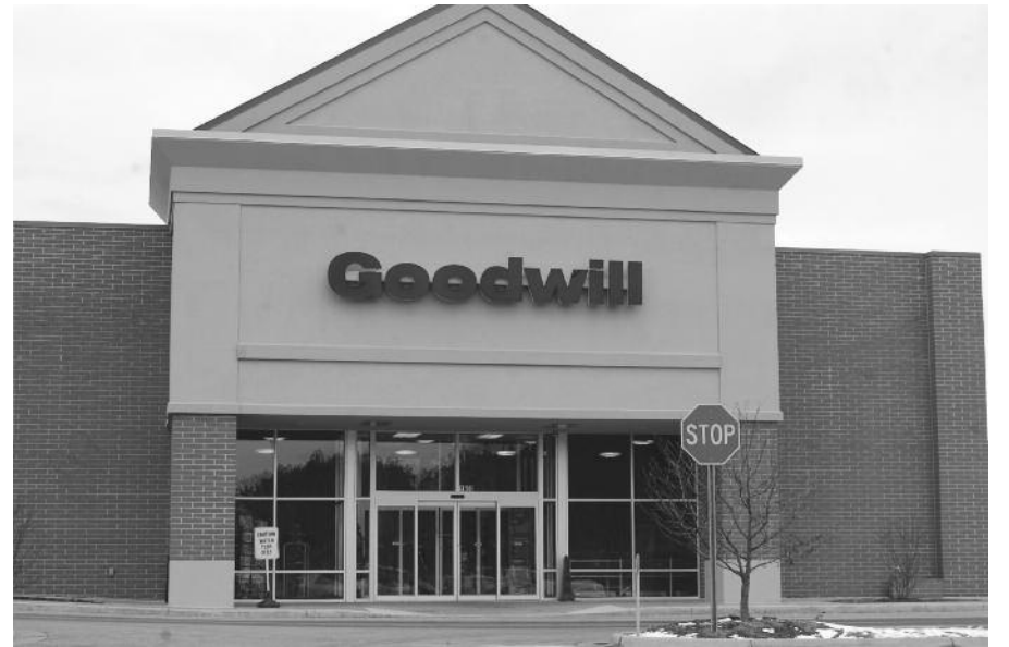
The 6,700 square foot Goodwill Retail and Donation Center in Petoskey is located at 1600 Anderson Road. PHOTO BY DAVE BARAGREY
