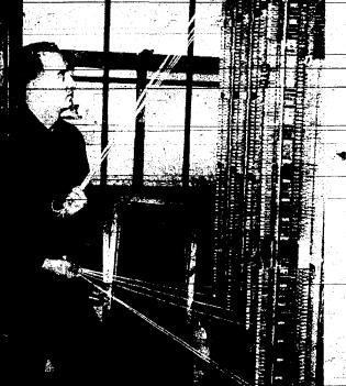
Me from A momement after this picture was snapped Graham this Michigan Bell workman yanked these cords at-visiting tached to the "heat coils" (tiny fuses) on the main frame which put the old office out of service.
