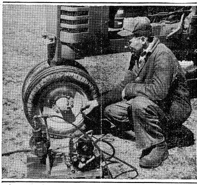
An old auto compressor comes in handy for a lot of farm jobs, accord-Ing to Wayne Williams, of Cedar Springs. He rigged his compressor to a small electric motor so it would be easy to use for spraying, dusting, applying fly spray, and cleaning small motors and farm seed tools, as well as for inflating tires. A pipe, bolted to the motor base, sets into two notched pieces of angle iron, which are bolted to the wooden base, to hold the portable motor in place.
