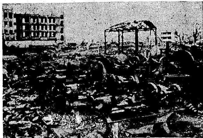
Home as well as factory industrial facilities felt the lash of U. S. air raids, with only the machinery standing in the ashes of this burned-out residential shop in Tokyo.
