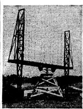
Close-up of the antenna of the first complete radar, installed "topside building at the Naval Research laboratory in the late 1930s. It is a so-called "dirigible" antenna, meaning it is so mounted that it can be turned to allow for around-the-com-pass search. This older model has recently been improved.
