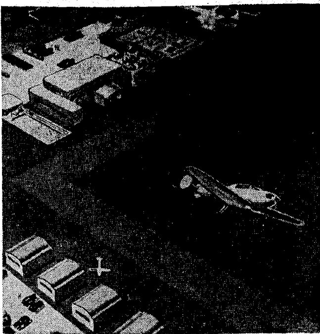
The Class 1 airport, known popularly as an "airpark," is designed for small private owner type planes up to 4,000 pounds gross weight. Fields of this class are designed to serve small communities, and as auxiliary airports in larger metropolitan areas. There are no paved runways, but landing strips with clear approaches must measure 1,800 to 2,700 feet long and 300 feet wide. Recreational facilities, such as parks, tennis courts and golf courses will surround the airpark in many cases.
