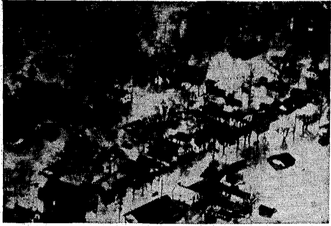
Flood waters spilling over the banks of the Ohio river and its tributaries again made thousands homeless and threatened war production. Aerial view shows Newton, Ohio, with a population of 2,000, isolated by the inundation.
