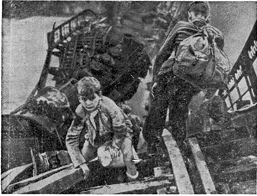
As train lies at bottom of Moselle river after plunging through wrecked bridge, French youth scramble over debris to salvage food from cars.
