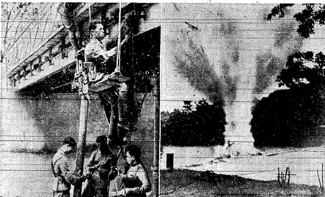
In the United States an ordinary railroad line would count its bridges and trestles by the scores or by the hundreds. In Java they are numbered in the thousands. Bridges are seen everywhere spanning rivers and ravines. And so, before Java fell to the invading Japs, the Netherlands East Indies mountain army became experts in demolition. At left they are seen as they mined a bridge. Right: A small pontoon bridge for infantry crossing is shown as it was destroyed by a well-placed shell.
