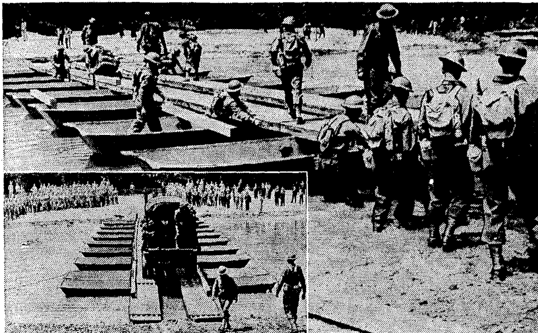
In a demonstration at Ft. Belvoir, Va., a motorized war-strength company of the Fifth Engineers dismounted from its trucks, unloaded equipment, and within 16 minutes constructed a 200-foot pontoon bridge strong enough to carry ammunition trucks. In picture at right, runways are laid across gunnels of light pontoons. Inset: Company "E" of the Fifth Engineers is shown crossing waterway on bridge.
