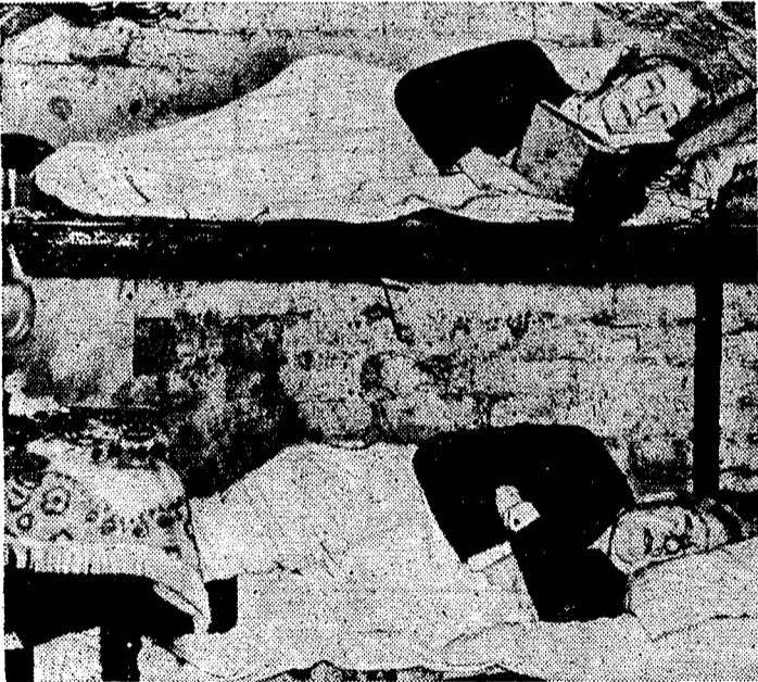
This aged couple spend the air raids in the de luxe shelter constructed in the basement of their Westminster borough home in London. The bunks upon which they rest were installed by the Westminster council which is providing them for all private shelters, to enable the populace to obtain their proper rest and curb "air raid nerves."
