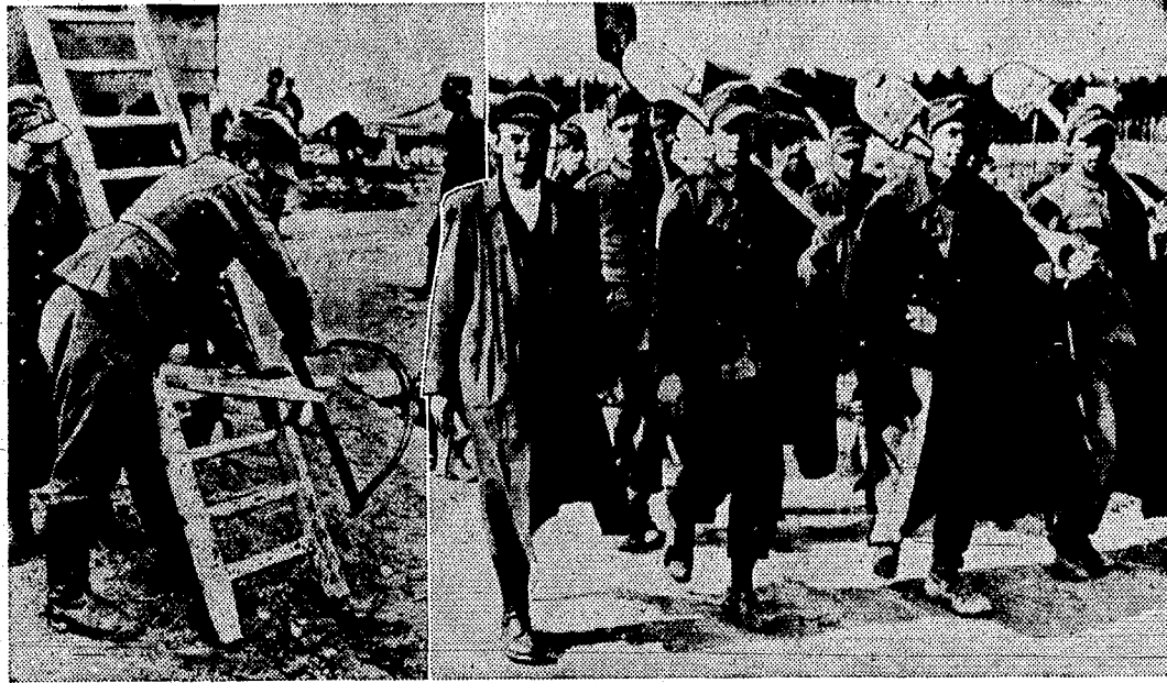
Polish soldiers who became prisoners of war when the Nazi blitzkrieg subdued their country are shown at work in a prison camp "somewhere in Germany." Many of them are at work constructing buildings to house prisoners, others labor with pick and shovel, thus releasing more manpower for German military duty.
