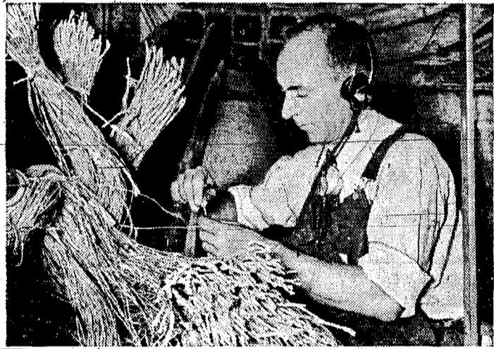
A hopeless tangle to the layman, intricate networks of underground wires are the plaything of telephone workers like this man. Every wire goes somewhere—and he knows where!
