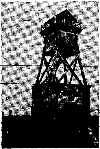
Lighthouse without seal. This North Carolina brick and wooden lighthouse, 140 years old, now stands embarrassed in a bog, far from water. But once Fort Caswell was an island and the old light with its gingerbread scroll work was a guide through the channel. The channel has long since been filled up but the durable old light still remains.
