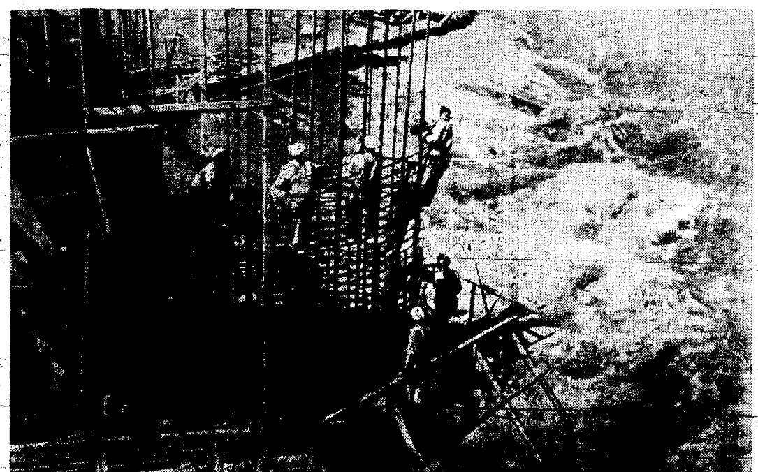
Army engineers are speeding the construction of the $32,400,000 Bonneville dam in the state of Washington. This interesting picture in which sky, water and steel meet shows workers erecting piers that will span the Bonneville river. This PWA project is a huge power, navigation and flood-control undertaking.
