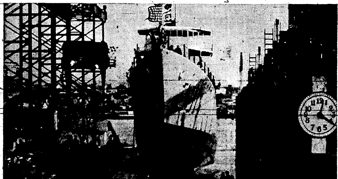
The U. S. S. Henley, launched recently at the Navy Yard, Mare Island. At the launching, the planned 1,500-ton destroyer was about 75 per cent complete and will be commissioned in the summer of this year, carrying a complement of 8 officers and 150 men.
