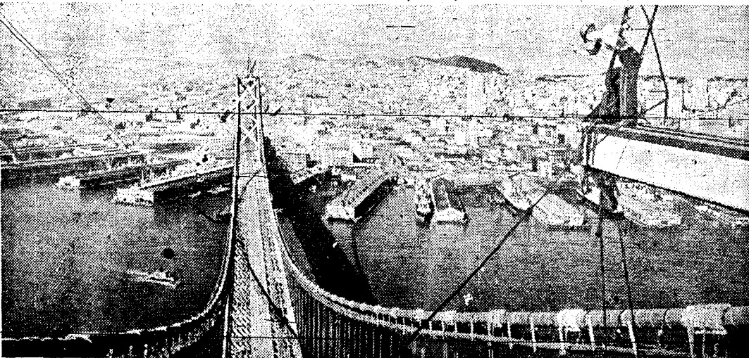
Automobiles will be passing over the San Francisco-Oakland Bay bridge by next November, engineers predict. This view shows the center lane with the floor steel entirely erected on the West Bay Crossing. The bridge, largest structure of its kind in the world, will cost $77,200,000 on completion.
