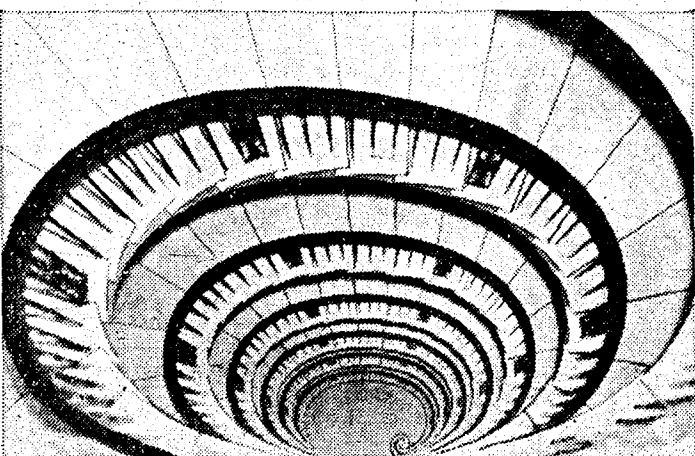
One of the remarkable features of the $9,740,000 Supreme court building, which was opened for the first time when the court convened for its autumn session, is the spiral stairway, of cantilever construction, shown in the above picture. The stairway, which seems to hold itself up without visible support, is fashioned of Alabama marble, like the rest of the building. Each tread extends into the wall on one side to the extent of 18 inches. There is no steel in the stairway, which is five stories deep. The picture was made from the top, looking down into the deep well.
